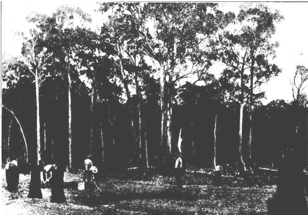
Making the Way to the Main Road – May 1930
